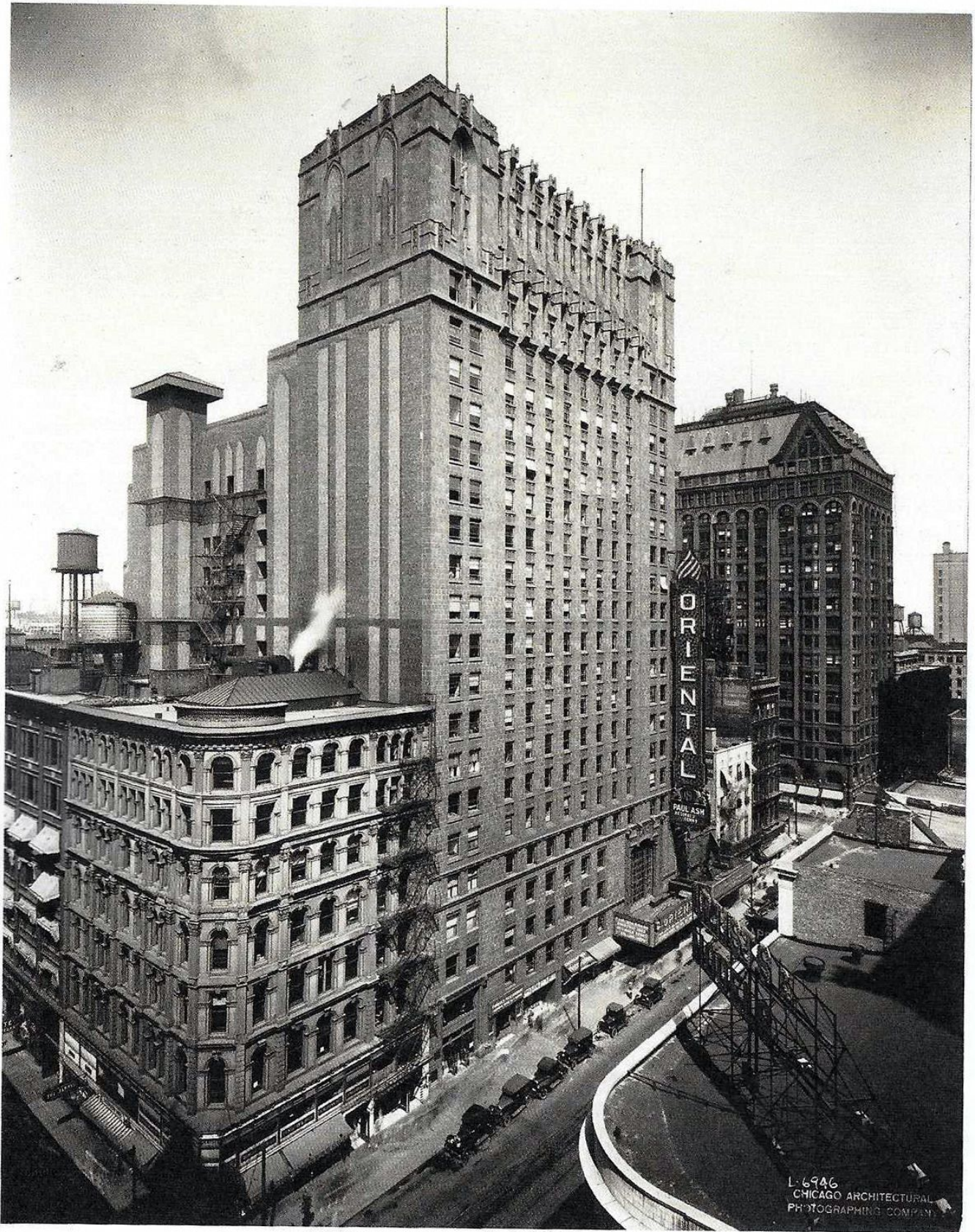
A third major multiple-use job in the busy year of 1926 was Chicago's Masonic Building and Oriental Theatre. The wary owners insisted that Rapp & Rapp give the building separate structural support in case the theatre failed and had to be torn out. (Chicago History Museum)
