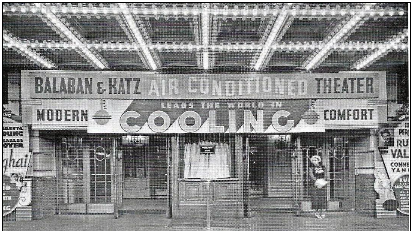
Note the air conditioning signs
